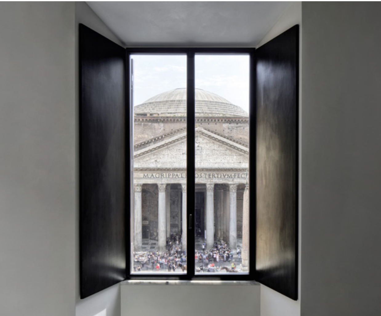
Double casement window with 47 mm sections constant around the perimeter and a central mullion of 62 mm.
