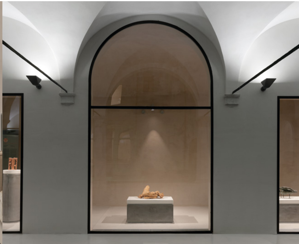
Fixed glass wall with constant profiles around the perimeter and the horizontal division.
