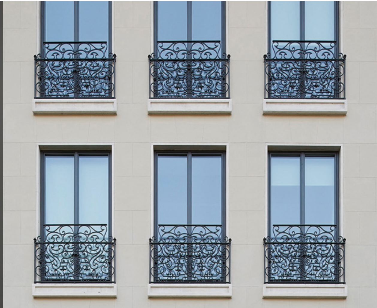
Double casement windows with constant 62 mm sections, both around the perimeter and in the central mullion.
