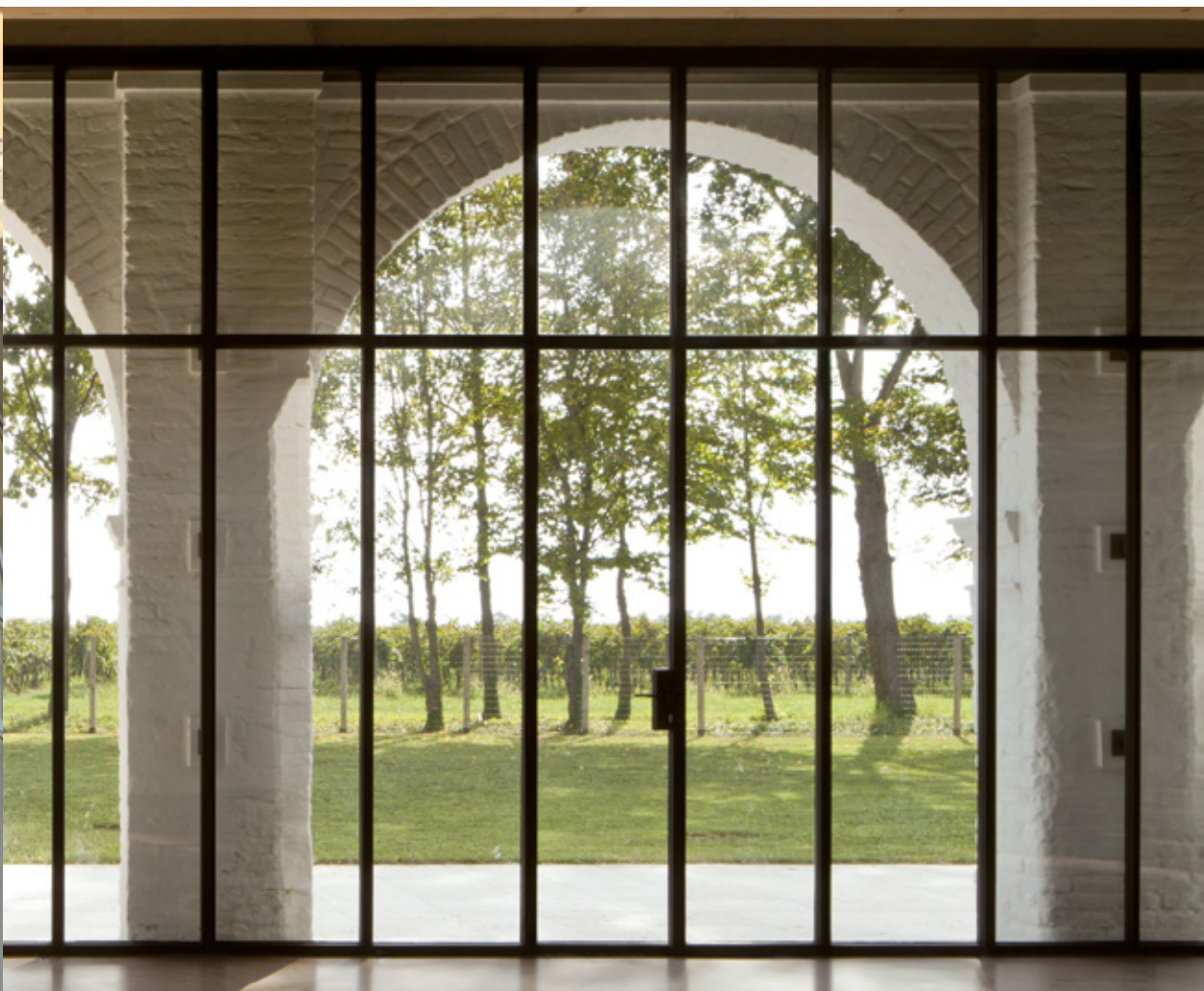
Window frame with coplanar glass panes and undifferentiated profiles between fixed and opening sections, making the openings imperceptible. Variant 2 of OS2 for Secco-type frames.
