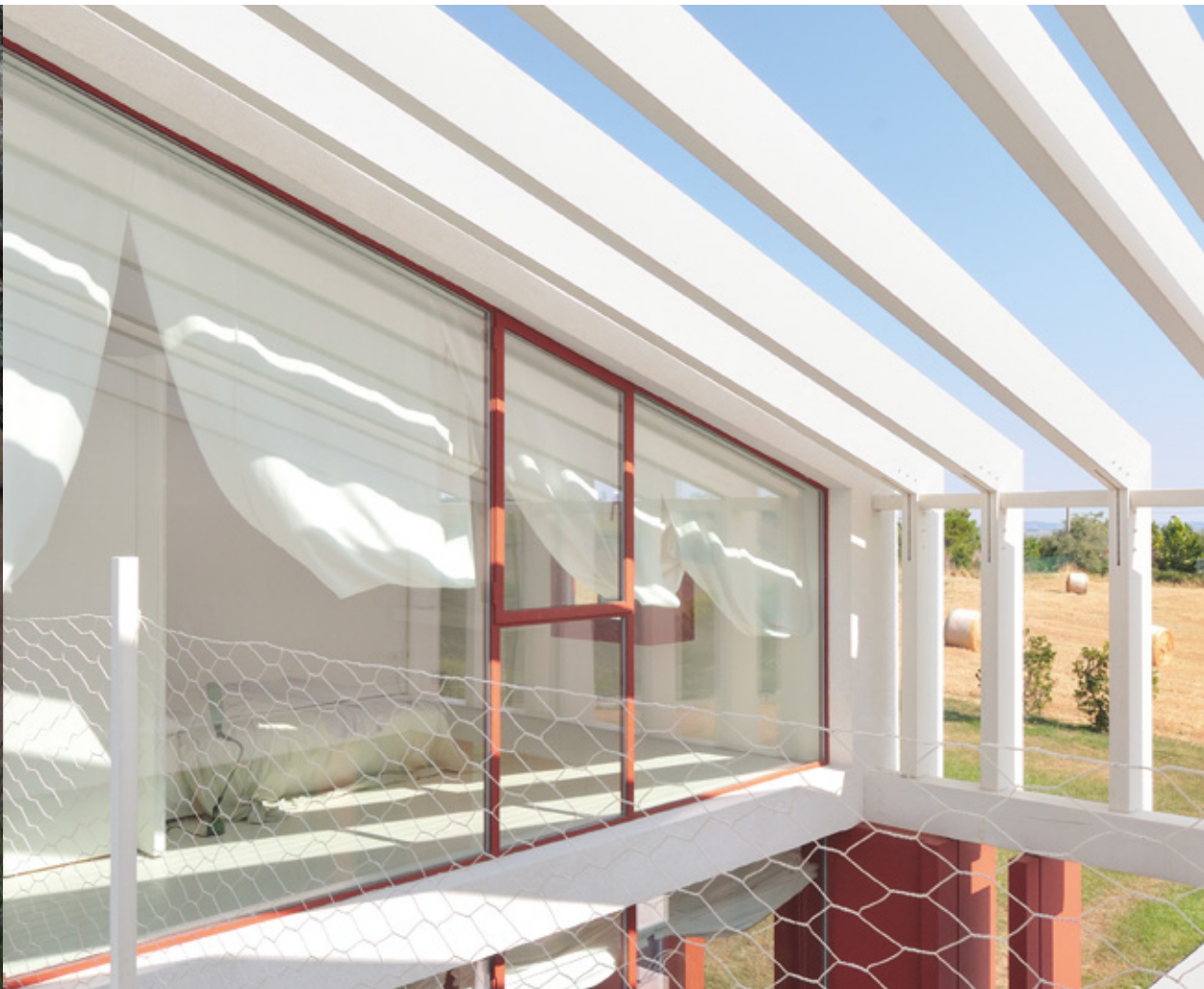
Single-leaf window with consistent joints around the entire perimeter, including the fixed bottom section.
