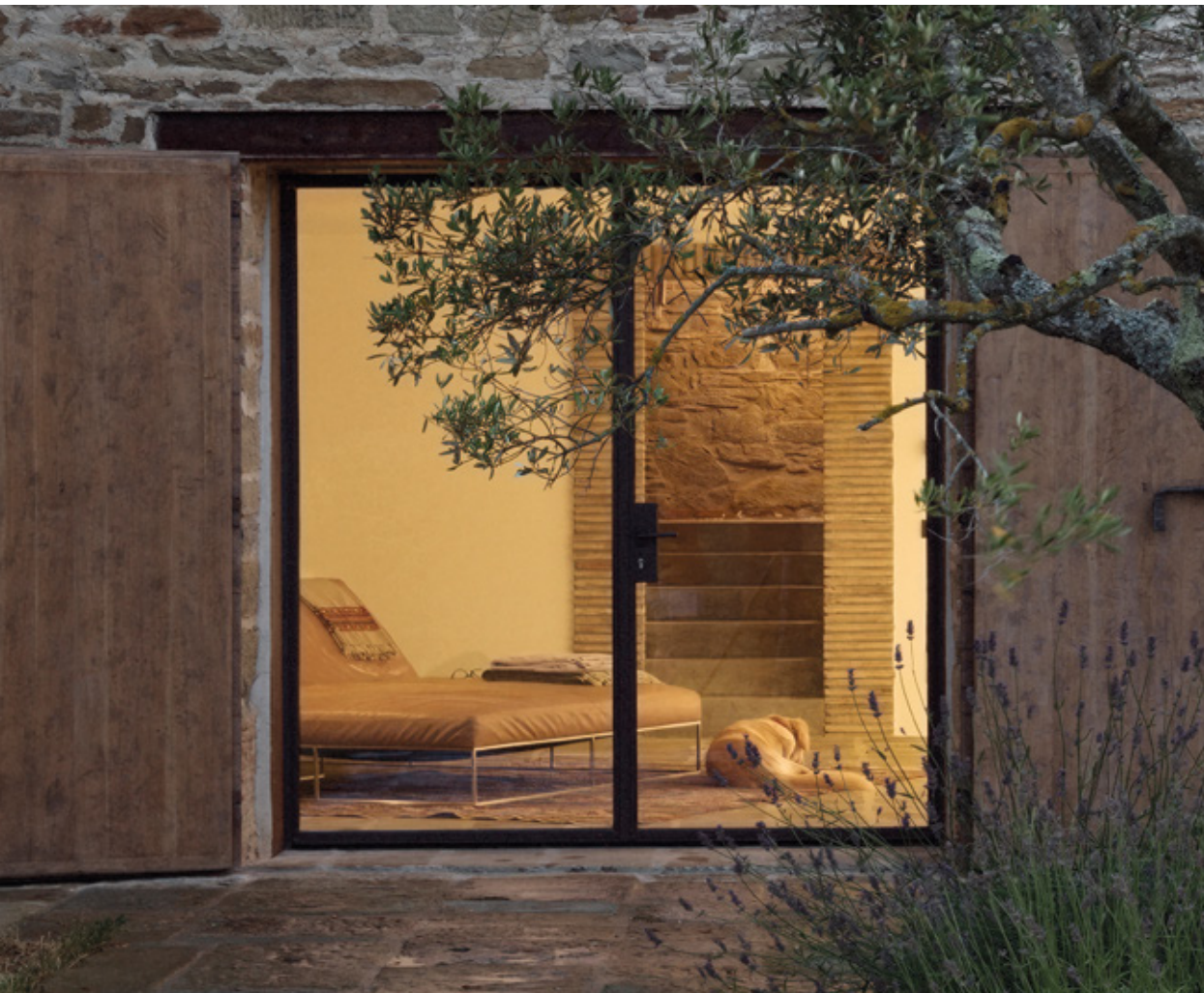
Double-leaf door with constant profiles, including the central mullion and floor section.
